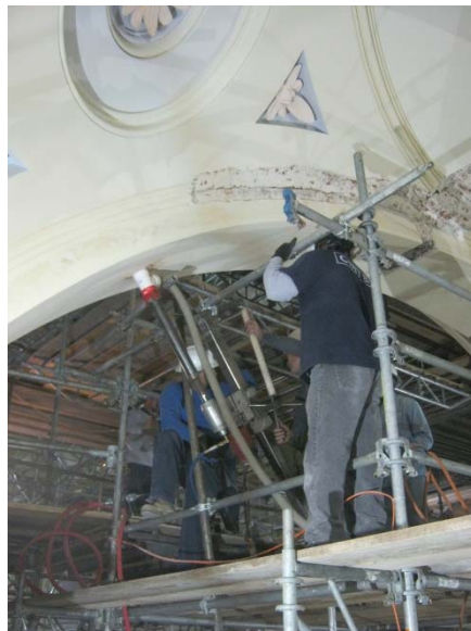
Figure 16. Application of Cintec wall anchors for brick masonry arch repair.
