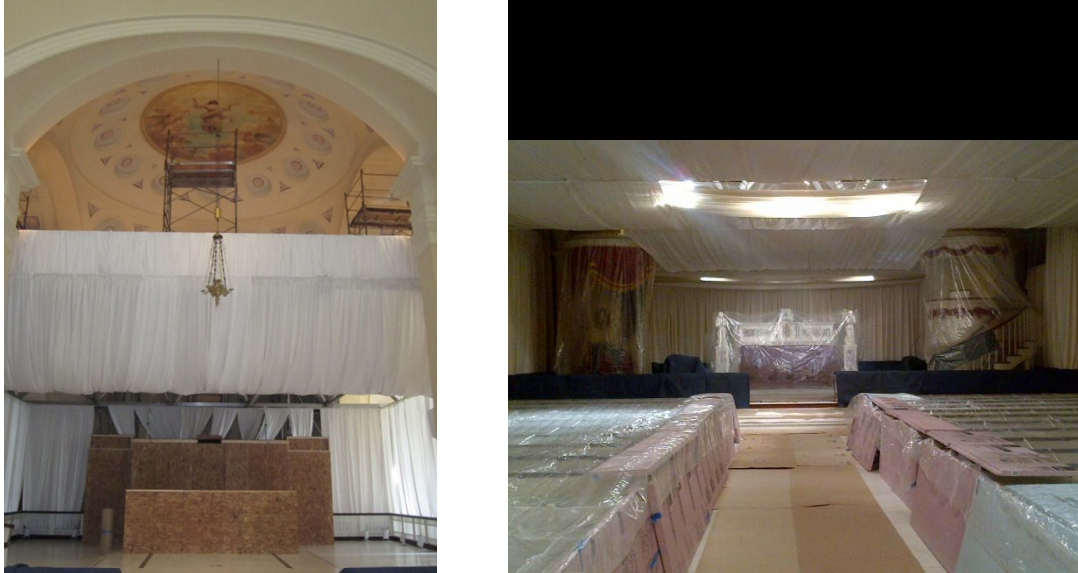
Figure 11. Finished truss draping and protection during construction.
