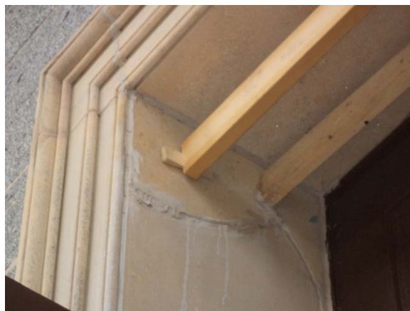
Figure 21. Marble door surrounds stone repair.
