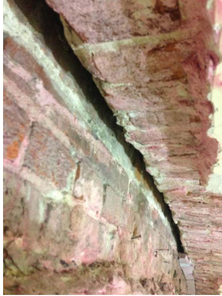
Figure 17. Masonry separation at brick dome connections to barrel vaults.
