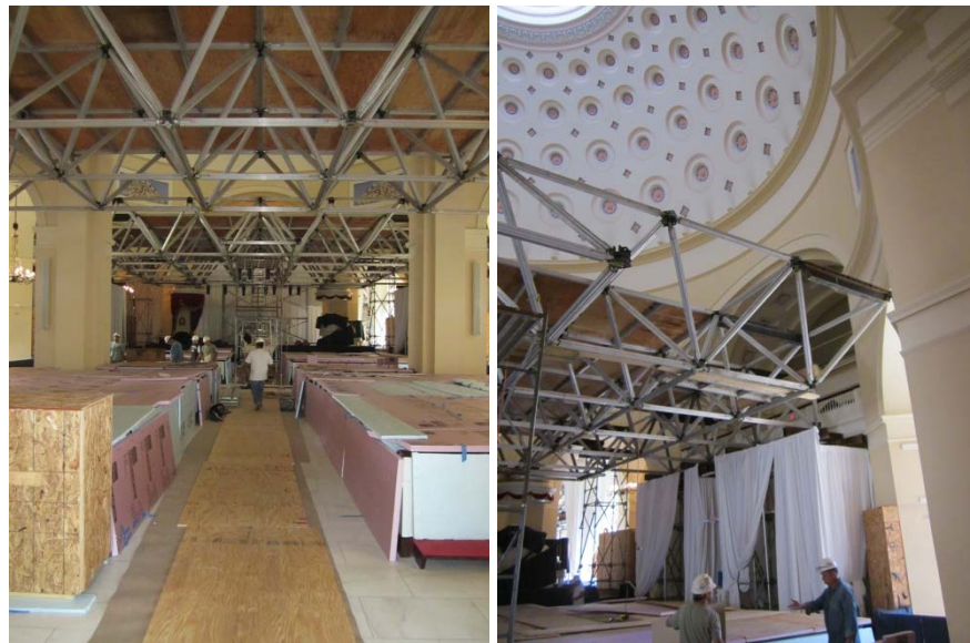
Figure 10. Truss scaffolding erection over pews and main worship space.
