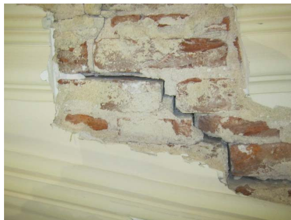
Figure 23. Cornice plaster repair at brick masonry arches.
