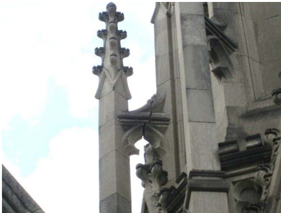
Figure 10. Broken tertiary pinnacle.
