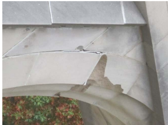
Figure 9. Damage at Apse buttress flier near pier.
