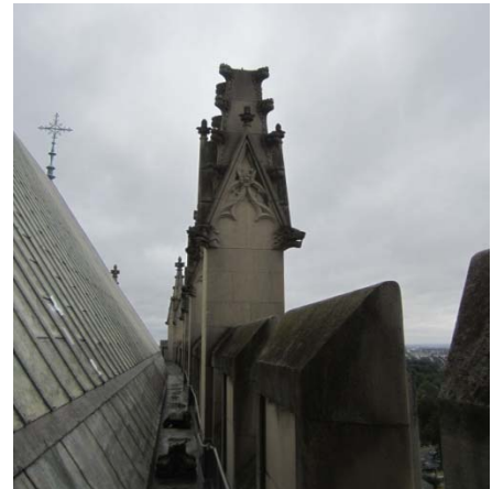
Figure 7. Broken pinnacle.
