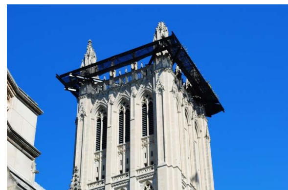
Figure 4. Platform and temporary protection at the Central Tower.
