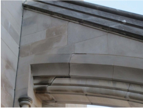
Figure 8. Damage at Apse buttress flier near Apse wall.
