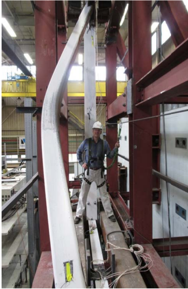
Above: A buckled HSS brace after testing in a full scale concentrically braced frame.
