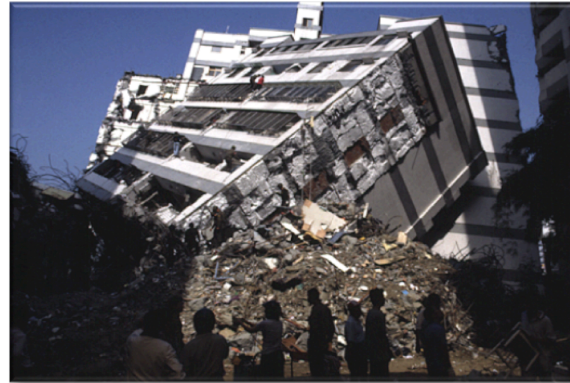
Figure 3. A lack of knowledge about existing vulnerable structures throughout the U.S. and around the world challenges our ability to develop resilient communities.
