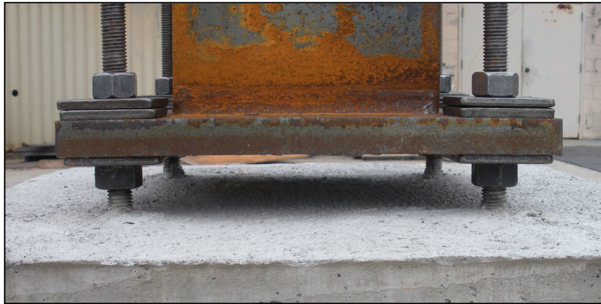
Figure 3.6 – Leveling (setting) nut detail
