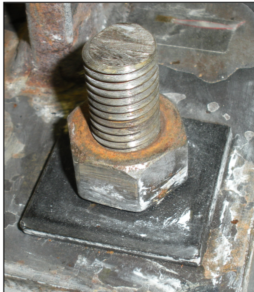
Figure 3.7 – Detail of anchor rod nut and washer assembly
