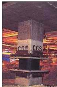
Figure 2: Typical Base Isolator
