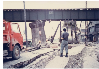
Figure 7. Tilted pier of Shinanogawa Bridge (Photo by Watanabe)
