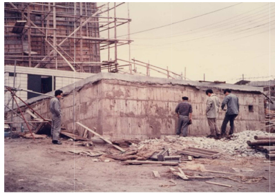
Figure 5. Uplifted sewage tanks (Photo by Watanabe)
