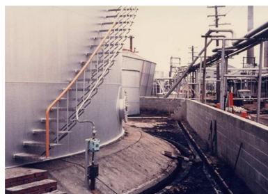
Figure 3. Settled and tilted oil tanks (Photo by Watanabe)
