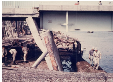
Figure 6. Tilted abutment of Yachiyo Bridge (Photo by Watanabe)
