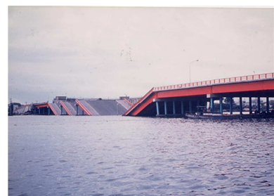
Figure 4. Collapsed Showa Bridge (Photo by Watanabe)
