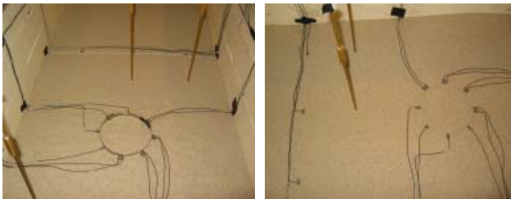
Figure 3.16 Bender layout (L: benders in placement and R: after completion)
