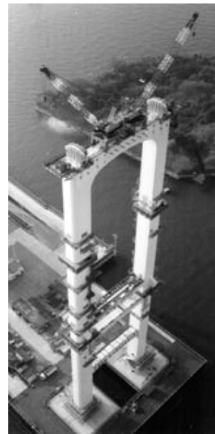
Figure 1.2 Rainbow Bridge Tower While under Construction.
