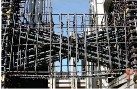
Fig. 1. Reinforcement detailing in diagonally reinforced coupling beam
