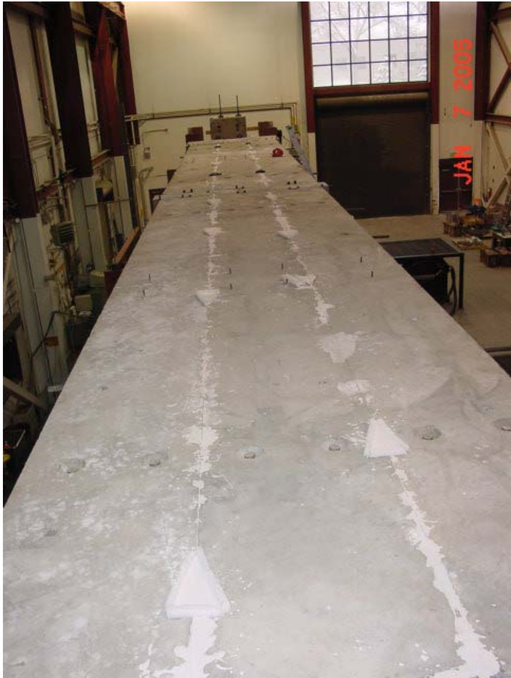
Figure 5-36: Superstructure after pouring of grout and hydrostone.
