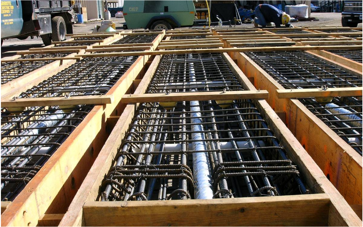
Figure 5-3: Superstructure beams prior to placement of concrete
