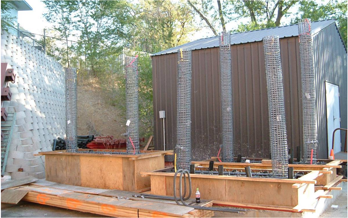
Figure 5-7: Column reinforcement cages after placement in footings.
