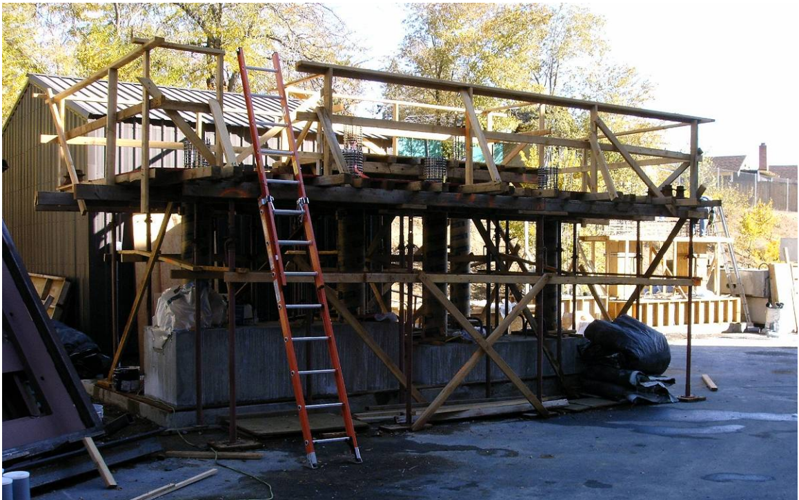
Figure 5-10: Completed working platform and installed sono-tubes.
