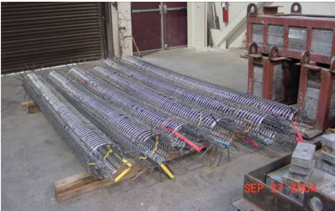
Figure 5-6: Column steel cages prior to placement in footing cages.
