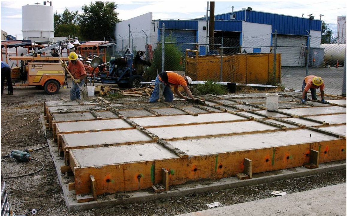
Figure 5-4: Placement of concrete for superstructure beams.
