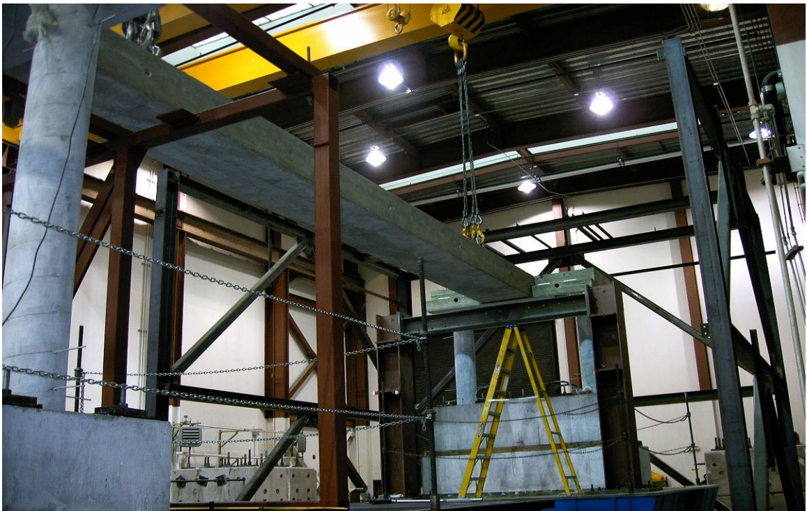
Figure 5-31: Placement of superstructure beams.
