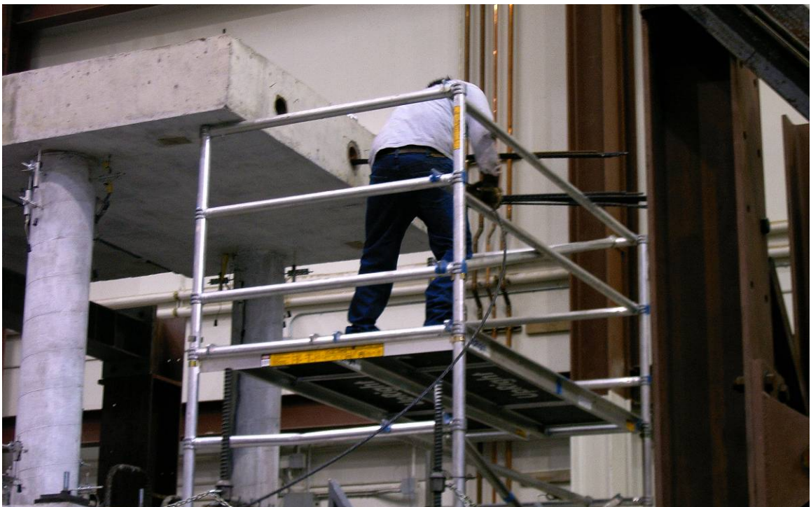
Figure 5-38: Longitudinal post-tensioning of superstructure beams.
