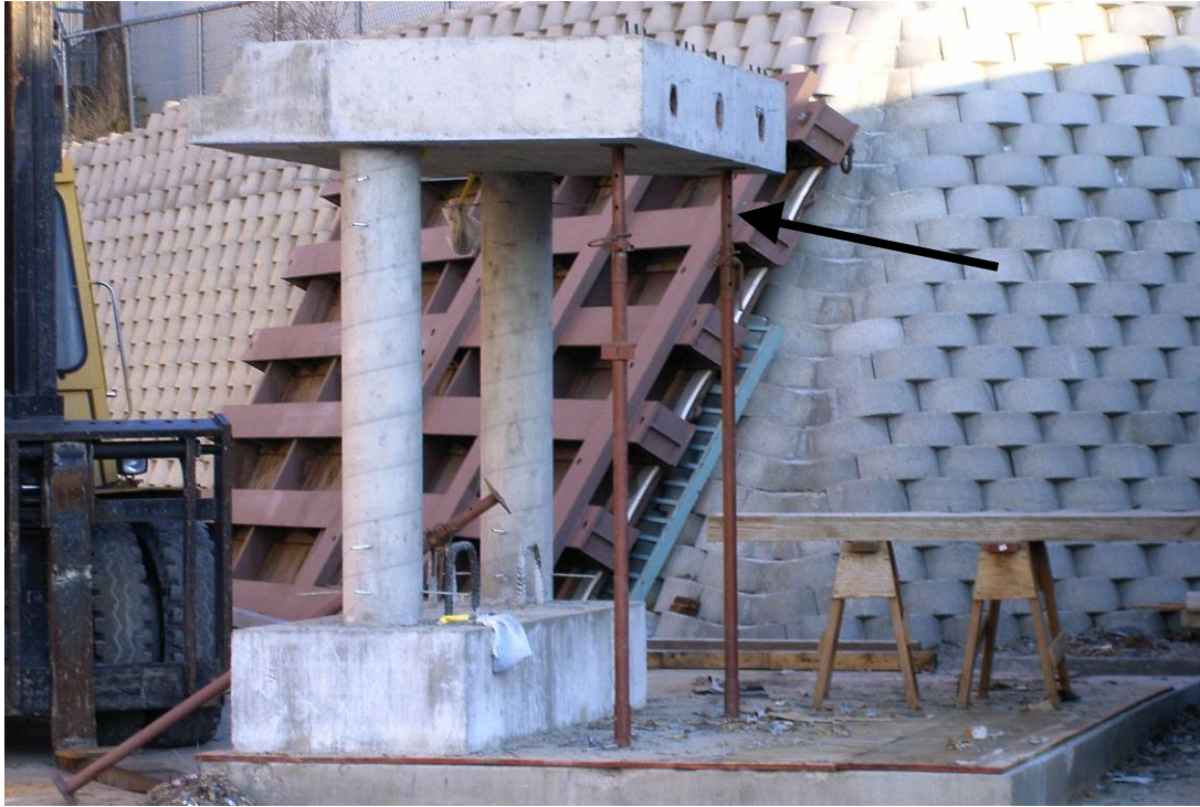
Figure 5-23: Bracing of cantilevers of bents 1 and 3.
