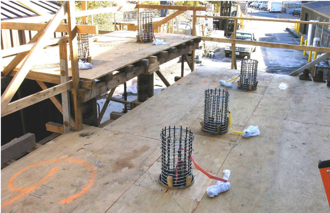
Figure 5-11: Top of working platform prior to pour of concrete for columns.
