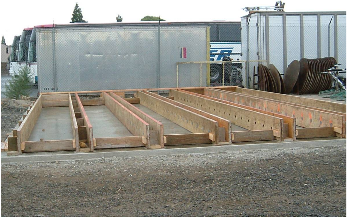
Figure 5-1: Off-site formwork for superstructure beams.
