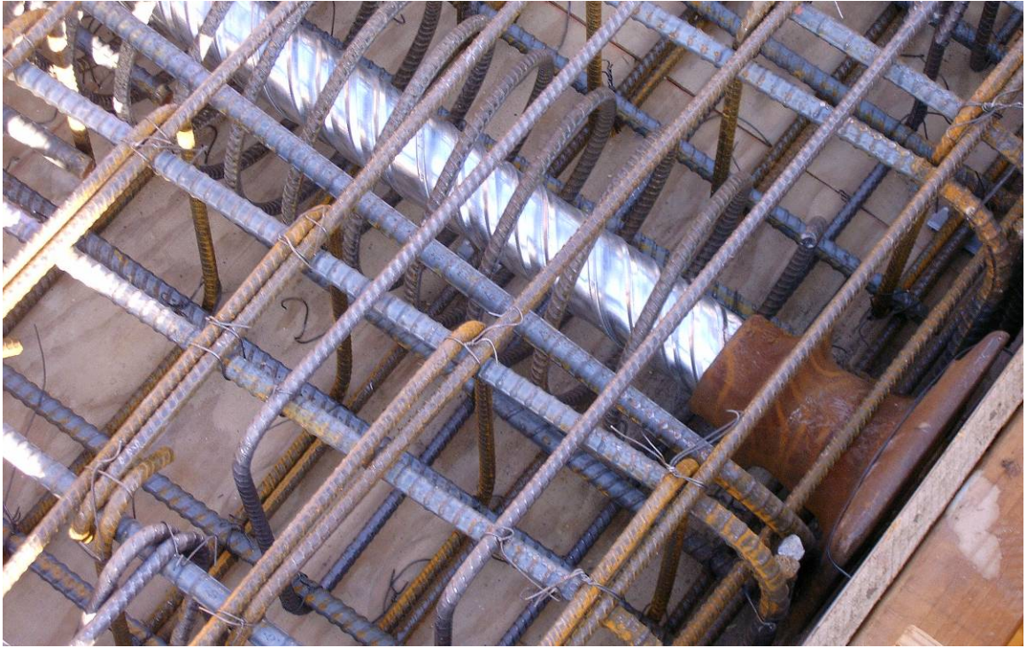
Figure 5-15: Installation of anchor and rebar spiral for post-tension anchorage.
