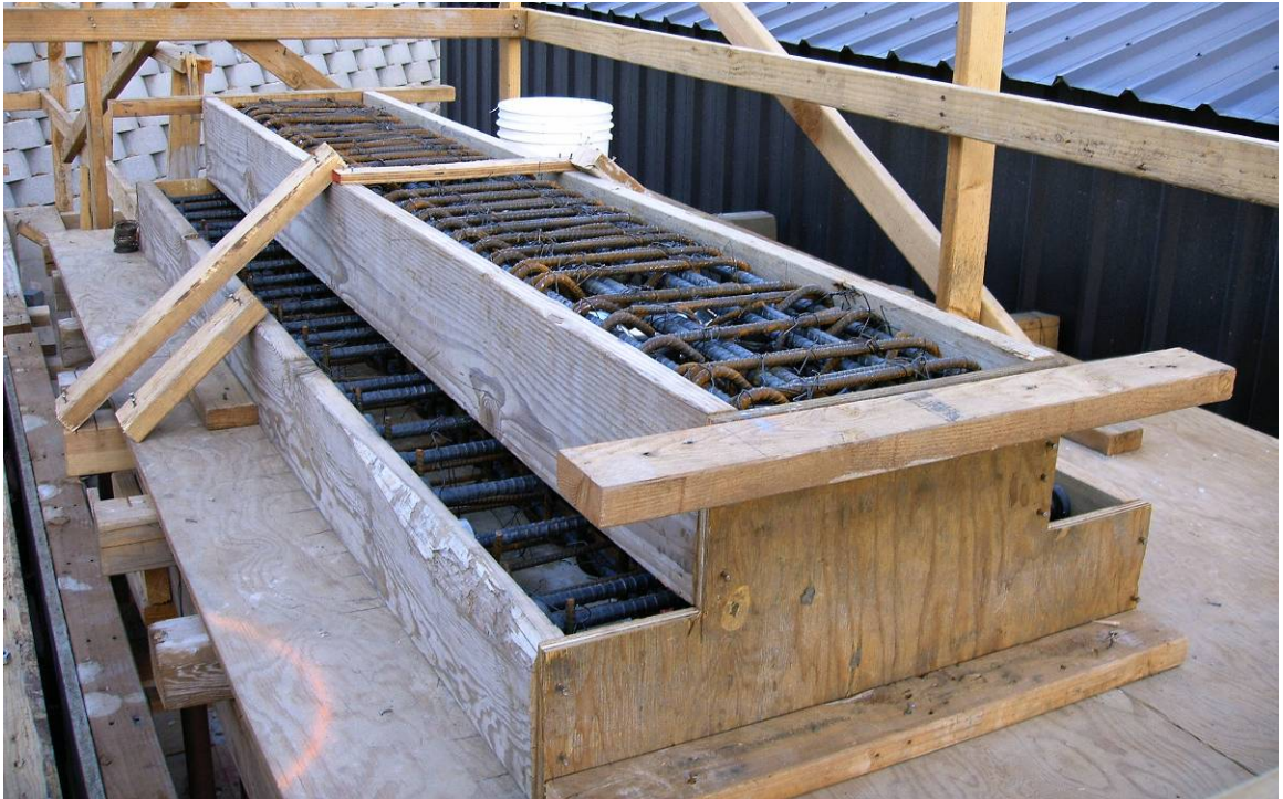
Figure 5-16: Formwork for bent-2 cap beam after assembly of cages.
