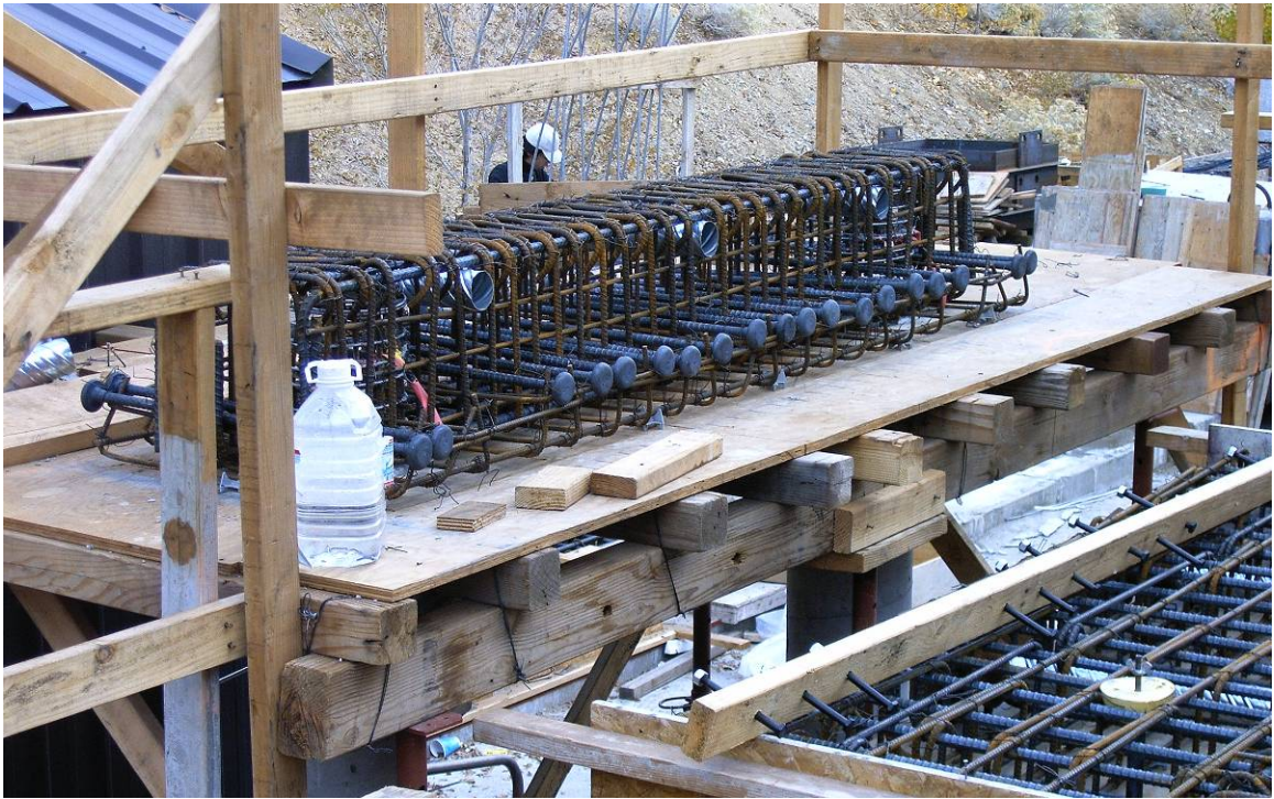
Figure 5-13: Assembly of reinforcement cage for cap beam of bent-2.
