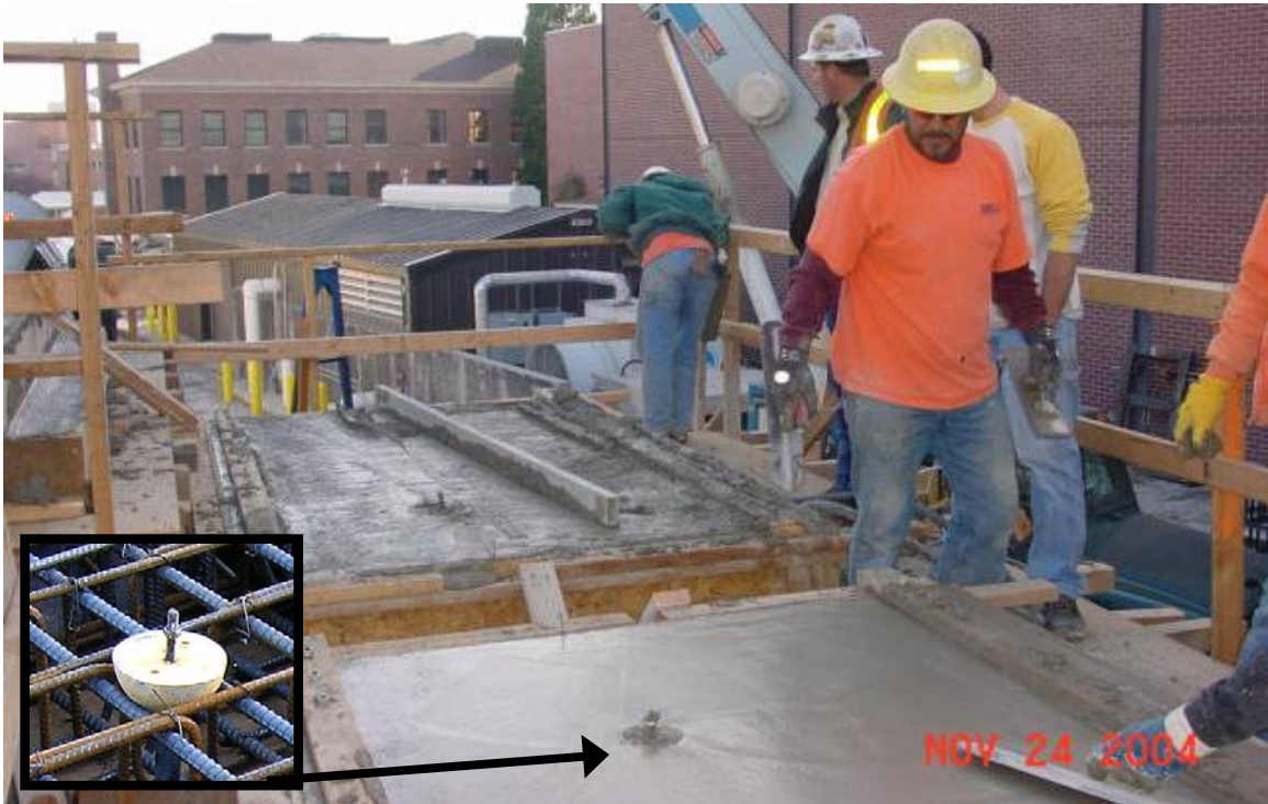
Figure 5-17: Placement of concrete for cap beams/cantilevers.
