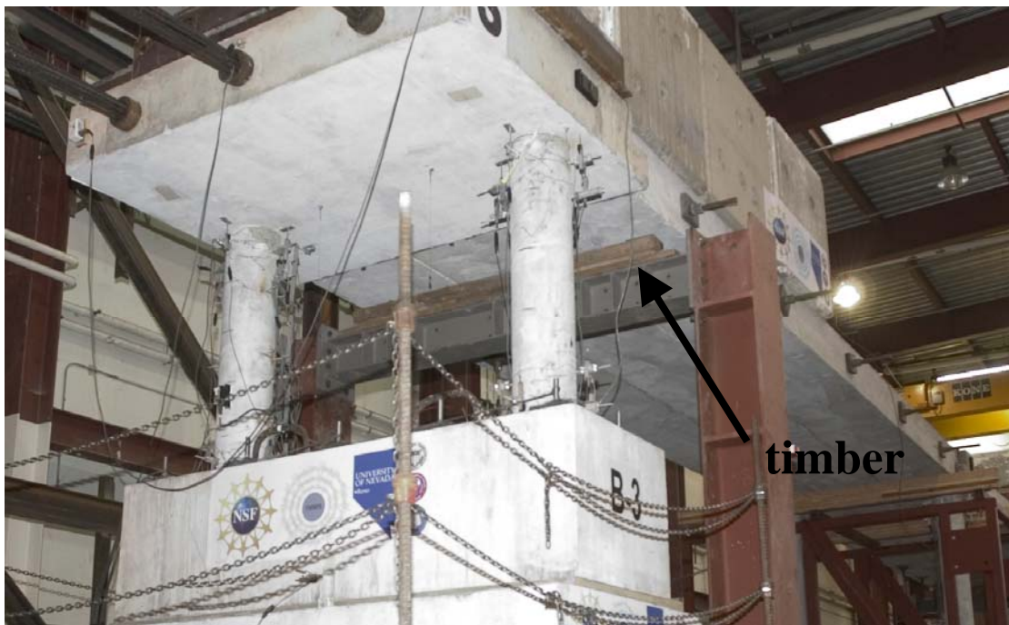
Figure 3-12: Photograph of shear bent 1 safety frame with timber on top.
