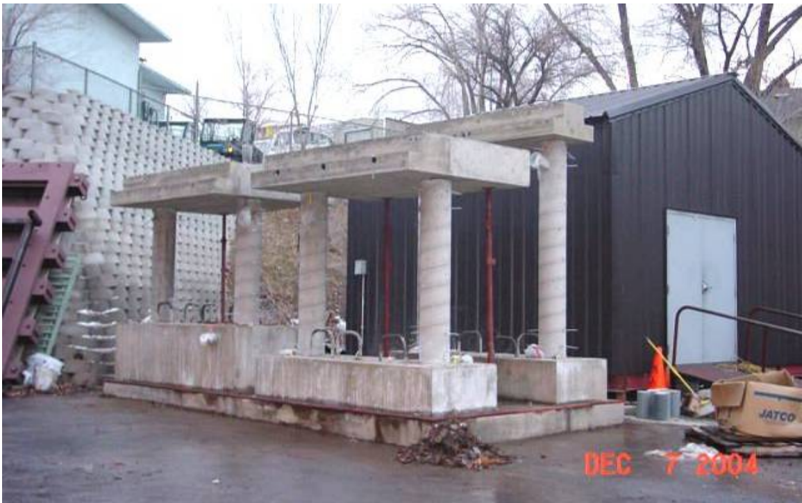
Figure 5-18: Completed bents 1 through 3 after removal of formwork.
