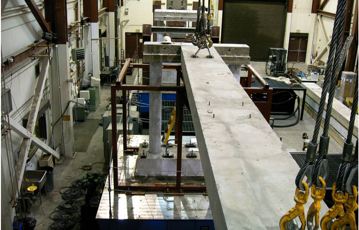
Figure 5-30: Lowering superstructure beams on to ledges.
