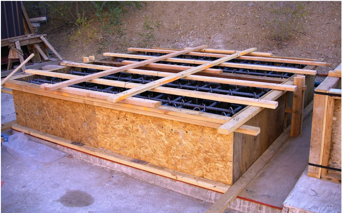
Figure 5-20: Completed formwork for spacer blocks prior to placement of concrete.
