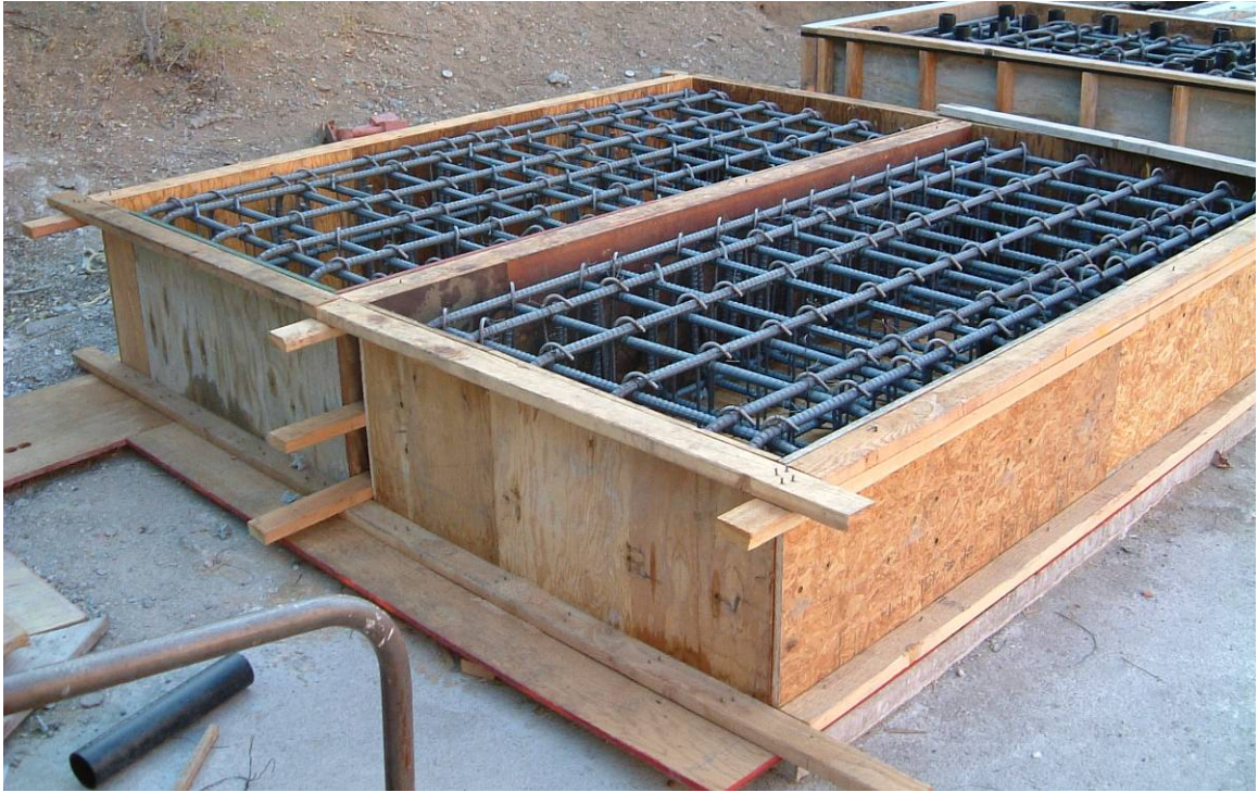
Figure 5-19: Reinforcement cages for spacer blocks.
