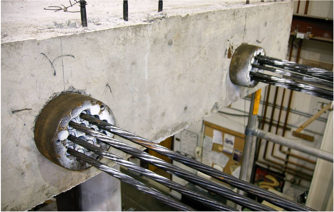
Figure 5-39: Collars and post-tension strands after longitudinal post-tensioning.
