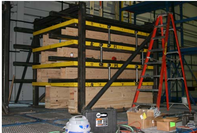
(a) completion of erection of mass simulator
